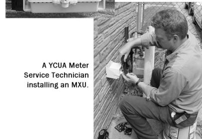
A YCUA Meter Service Technician installing an MXU.
